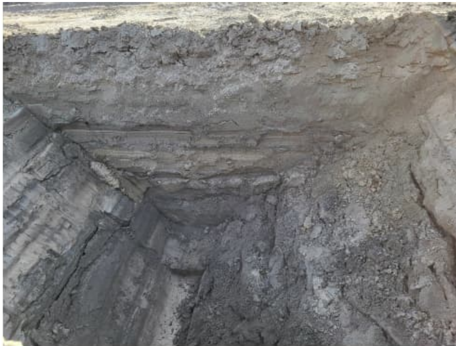
Photograph 3: Workable conditions following dewatering operation, test pit excavated to 5.2 m depth
