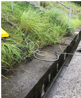
Photo 1: Leachate of perched water from berm of embankment
