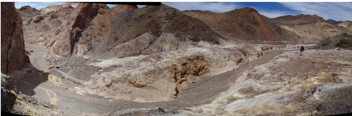
Figure 1: Photo of the Upper Castaño Viejo Dam site. Extreme left: starter dam location. Center: sliding surface. Extreme right: decant pond location.
