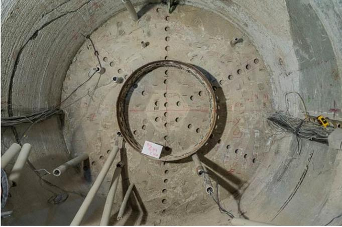
Figure 6. State of the barrier in the final dismantling. The location of the samples extracted from this section can be noted.
