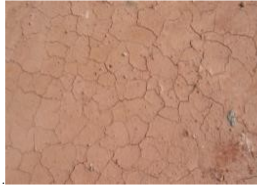
Figure 1. Landfill cover soil with cracks.
