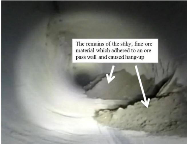
Figure 1. The photograph shows the inside of an ore pass (looking down) once a hang-up had been dislodged by intervention. The remains of the sticky, fine particles which adhered to the ore pass wall are clearly visible. The ore pass is circular in section with a diameter of 2.8 m and its inclined at 70° above the horizontal. The ore contains particles as large as 1.2 m, although larger particles do not adhere to the ore pass wall so they are not present in the photo.
