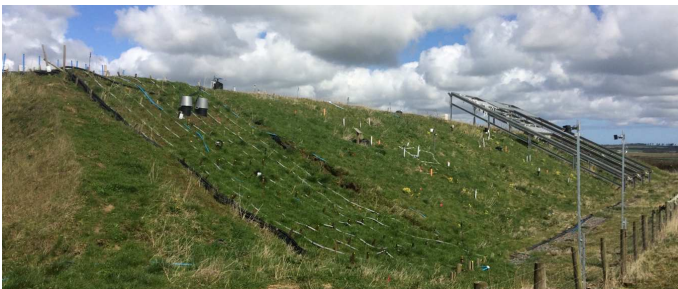
Figure 1. BIONICS Full-scale embankment test site, Newcastle University.
