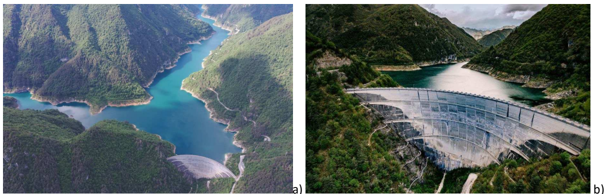
Figure 1: a) Aerial view of the dam and the Valvestino lake; b) Valley facing of the dam.
