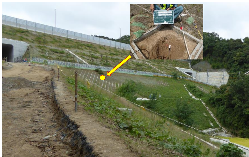
Photo 1: Embankment for field measurement.
