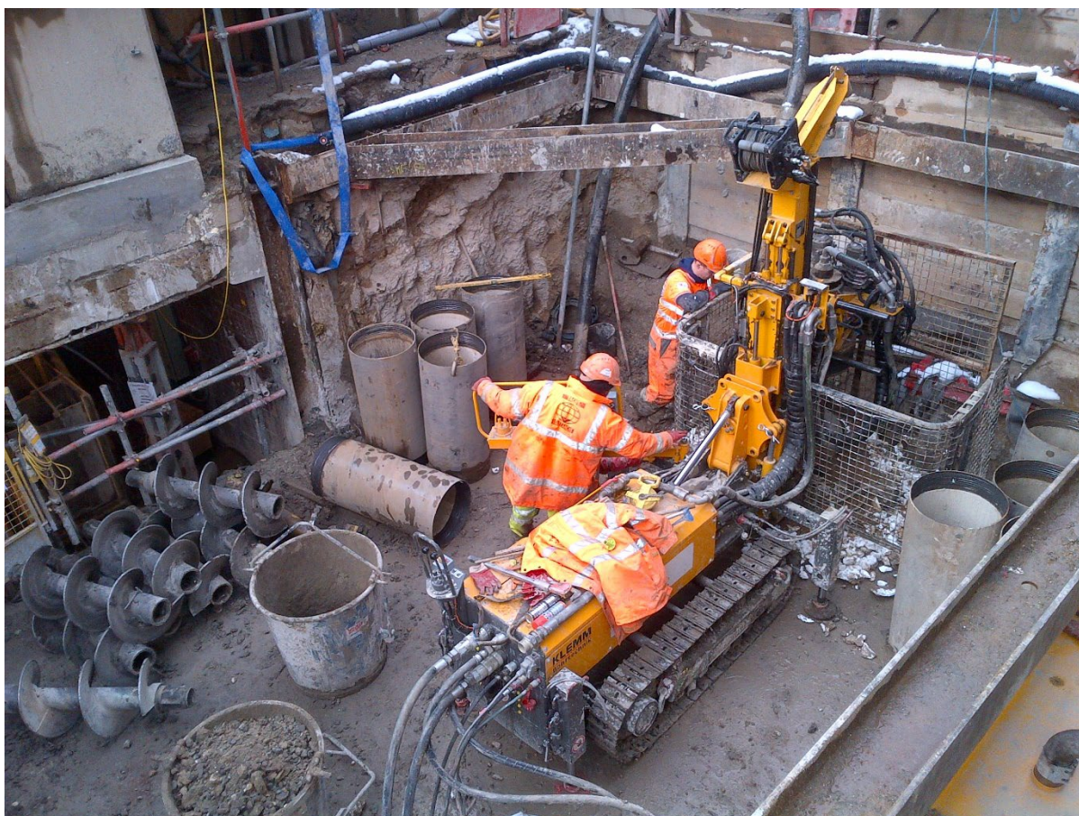
Figure 2: Piling for grout shaft in front of No 2 Stratford Place.
