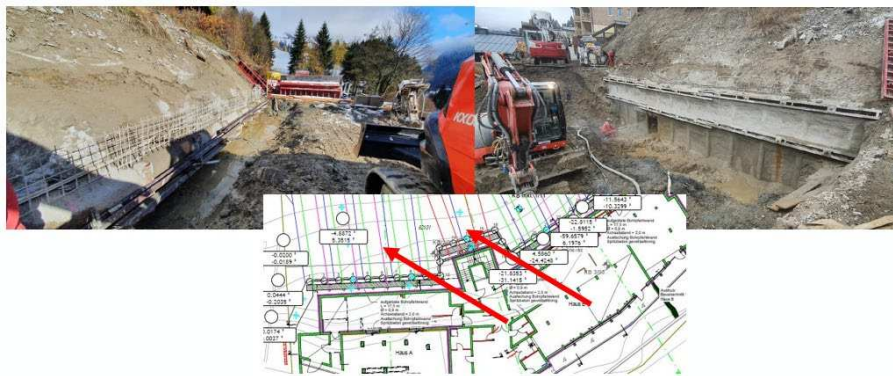
Fig. 19: Excavation and micro piling works November 2021
