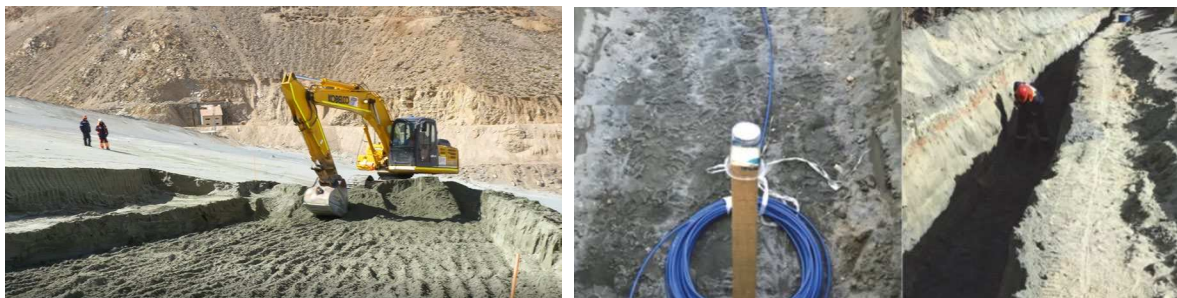
Figure 7: Maintenance of the dam and laying of Hydro&Geo strain sensing cable
