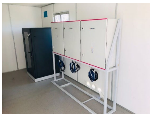
Figure 5: Air-conditioned control room: black cabinet with reading unit and accessories + three heating modules
