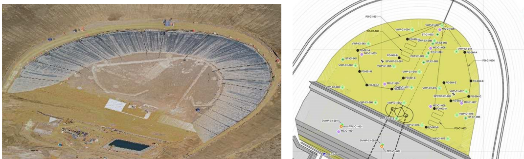
Figure 4: Top view of the first layer: 4 independent fibre optic cables
