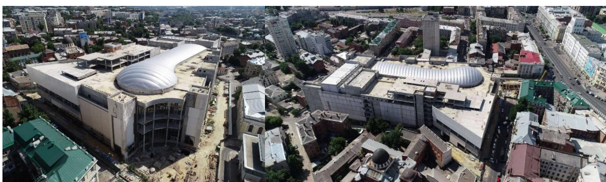
Figure 2: General views of the construction project (2020)
