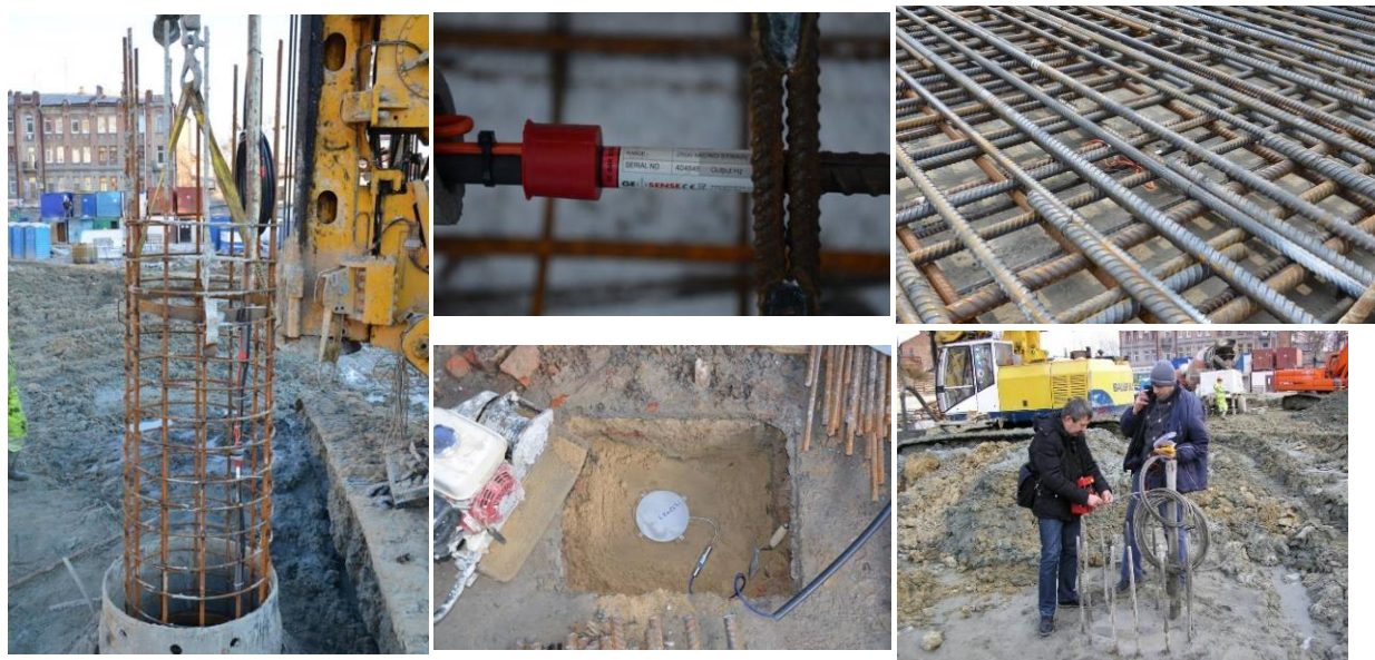
Figure 3: Installing different types of transducers and taking initial readings
