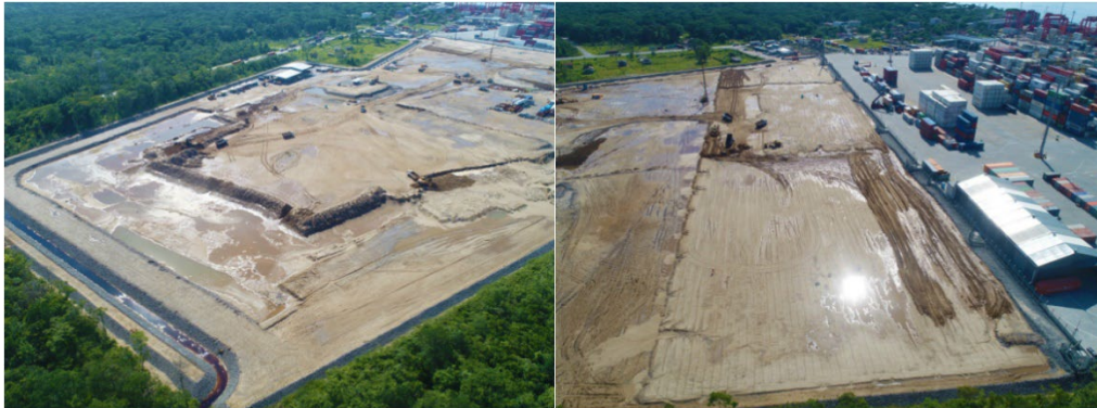
Figure 2: Aerial view of the port expansion area during overload landfill movement.
