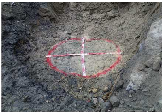
(a) Exposed of Jet Grouting column \phi=2.0 m
