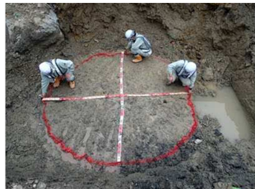
(b) Exposed of Jet Grouting column \phi=3.2 m
