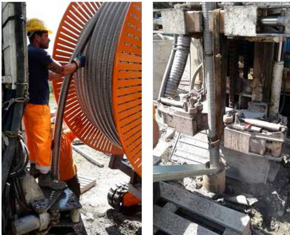
Figure 4. Installation of corrugated pipe.
