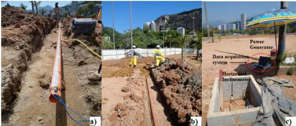
Figure 16. Tube installation: a) adhesive tape over FBG; b) ditch backfill; c) data acquisition system.
