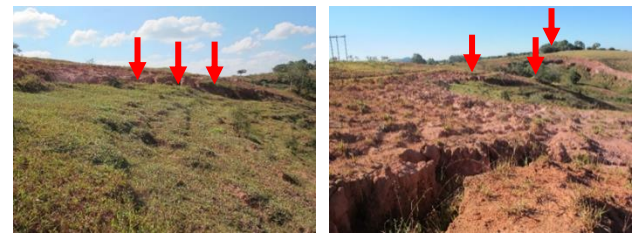
Figure 7. Part of the gully head: highlights for the “stair” formation on the ground.
