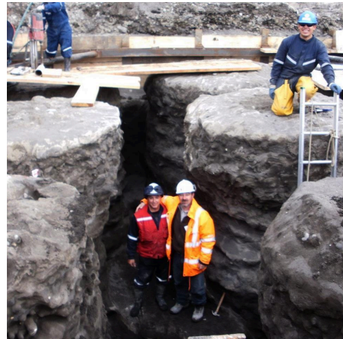
Figure 5. Exhumation of Jet Grouting Column in silty sands, Constitución (ref. Pilotes Terratest).
