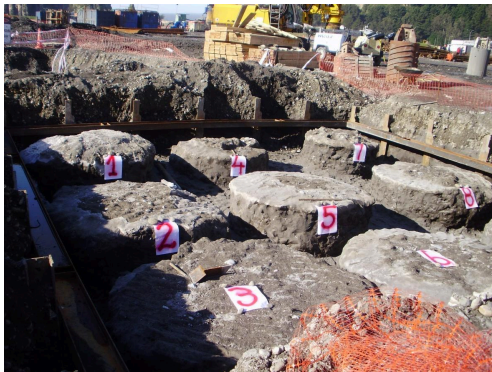
Figure 4. Exhumation of Jet Grouting Columns in silty sands, C (ref. Pilotes Terratest).
