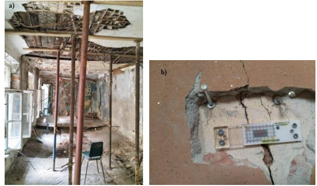
Fig.4. – View of a room with destroyed wooden floors (a) and a lighthouse installed on a crack for observation during geotechnical monitoring (b)
