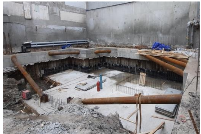
Fig. 11. View of a part of an arranged excavation with an angular spacer system
