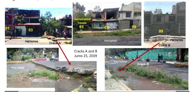
b) Condition of cracks A and B and adjacent houses on June 25, 2019. Figure 14. Condition of houses damaged by soil cracking.
