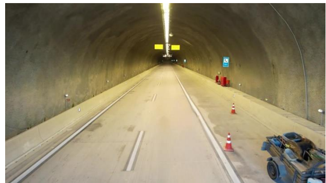
Figure 3 – Tunnel inner condition.
