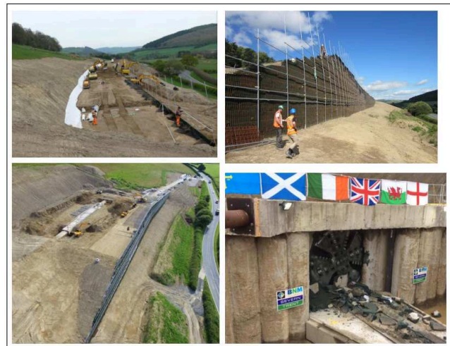
Figure 3. RSW Construction process and breaking through TBM – Elan Valley Bleddfa
