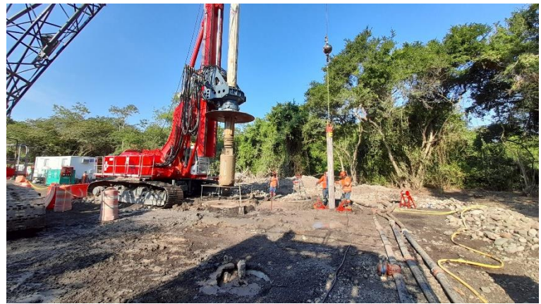
Figure 6. Drilling test and reaction piles.
