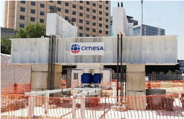
Figure 4. Reaction frame for unidirectional load test.
