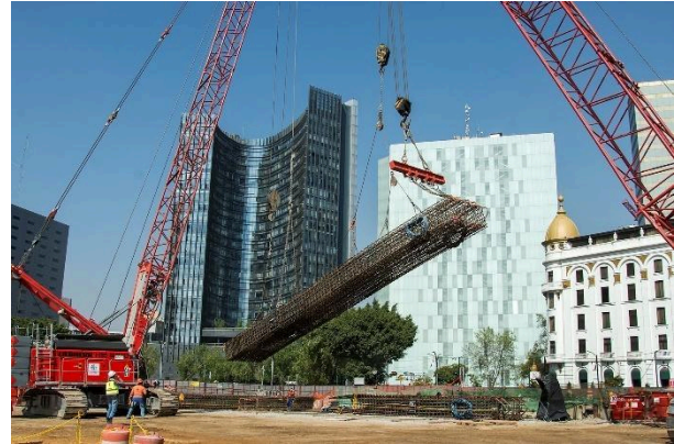
Figure 8. Lifting of reinforcement section with Osterberg Cells.
