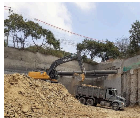
Figure 10. Screen of tangent piles and die-shot concrete wall.
