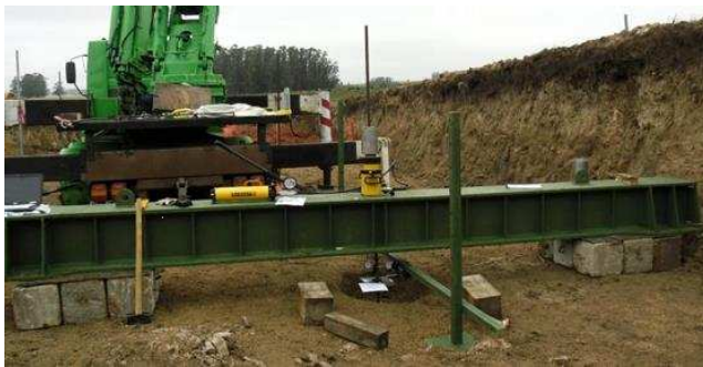
Figure 4. Reaction system for vertical anchor testing – Site 1.
