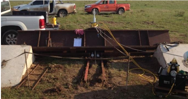
Figure 6. Reaction system for inclined anchor testing - Site 2.
