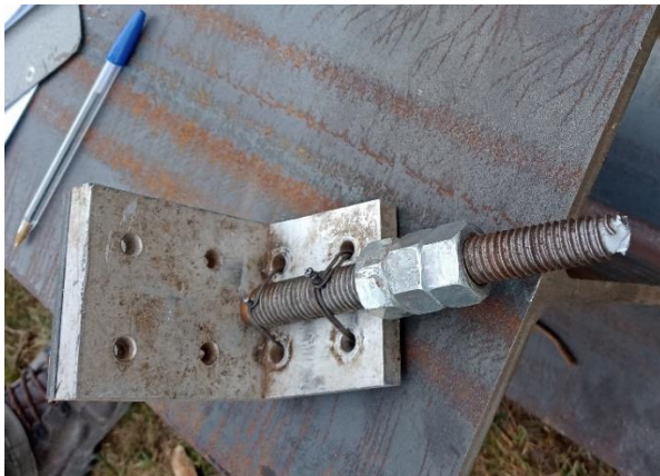
Figure 13. Anchor breakage due to steel creep – Site 4.
