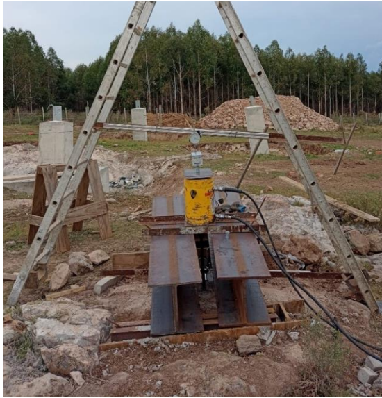
Figure 12. Anchor testing device for vertical anchors – Site 4.
