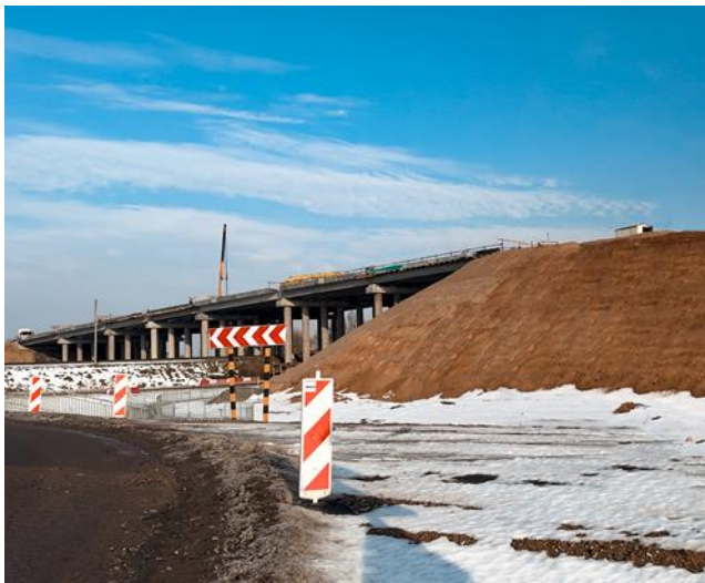
Figure 10. Reinforced embankment complete and overpass under construction.
