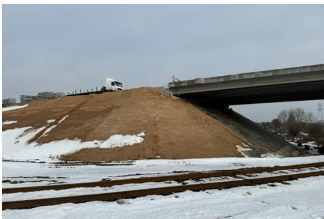
Figure 11. Constructed embankment.
