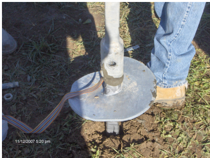
Figure.5.a. Typical preparation of lead section – extension connection
