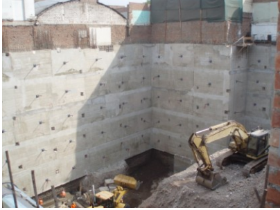
Figure 10. Seven level basement excavation in Lima, Perú.
