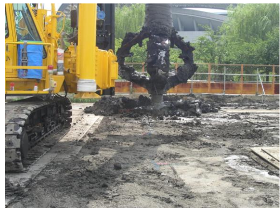
Figure 1. Columnar deep mixing method
