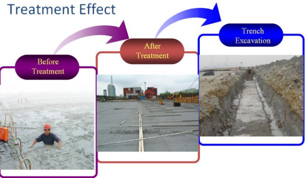
Figure 5. Photos of site condition prior and after HVDM.
