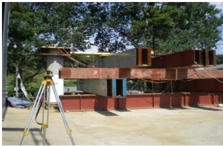
Picture 1. Lateral Load Test
