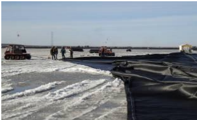
Figure 9. Deployment of a fabricated panel on the ice
