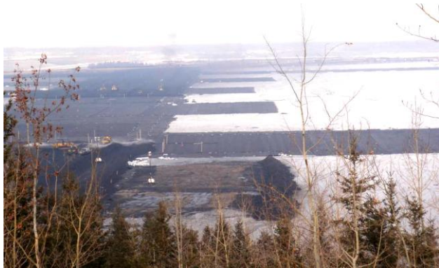
Figure 12. Extent of roads at end of construction in winter of 2010
