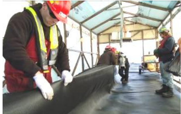
Figure 10. Field seams being sewn in the heated sewing trailer
