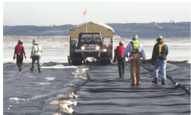
Figure 1. Preparing to sew a seam on the ice. Note stockpile of coke in the background.
