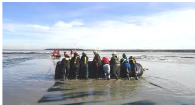
Figure 11. Last few panels placed before spring melting stopped on-ice activities
