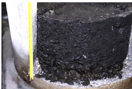
Figure 7. Exposed condition of aggregate after removal of section of test cylinder
