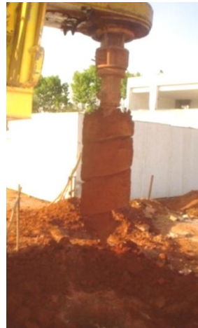
Figure 7. Column borehole execution.
