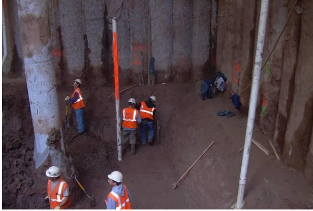
Figure 7. Excavation at full depth.
