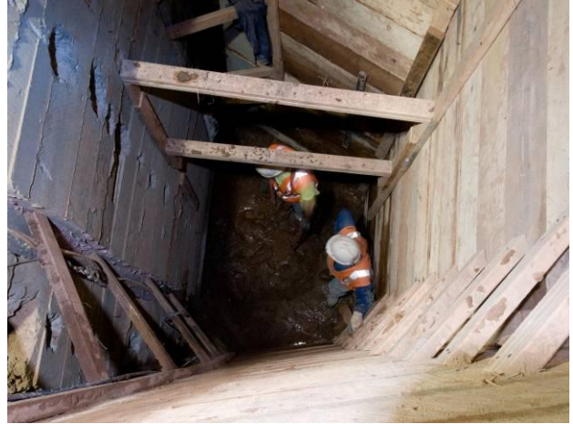
Figure 9. Hand excavated pit.
