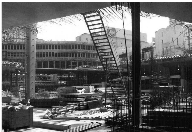
Figure 9. View from under beneath the ring slab.
