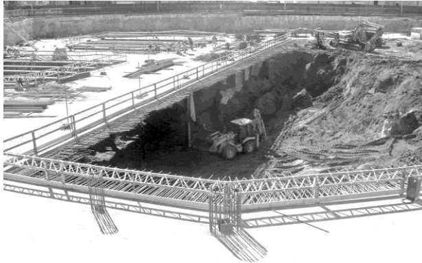
Figure 8. Excavation under the ring slab.
