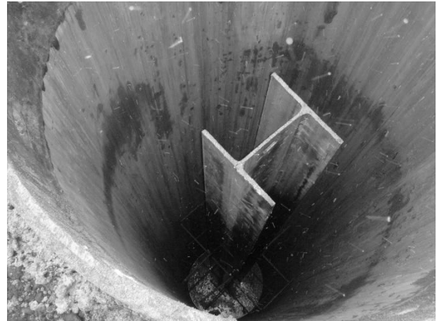
Figure 6. Pile with Steel Beam Profile
