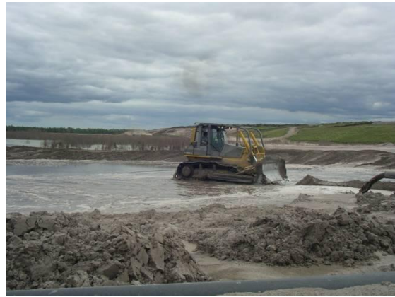
Figure 3. Compaction of coarse tailings by the cell method.
