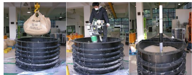
[1] Sand raining [2] 1 st Compaction [3] Pipe installation
