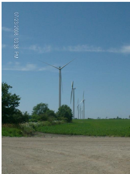
Photograph 1. Example of Wind Turbines already Erected
