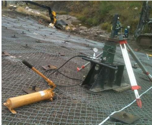
Figure 7. Soil nail pullout test setup
