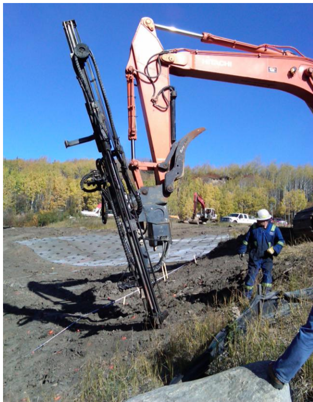
Figure 5. Percussion soil nail installation equipment.
