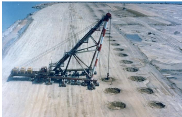
Figure 1. Giga-machine lifting a 172 tonne tamper at the Nice Airport (France).
