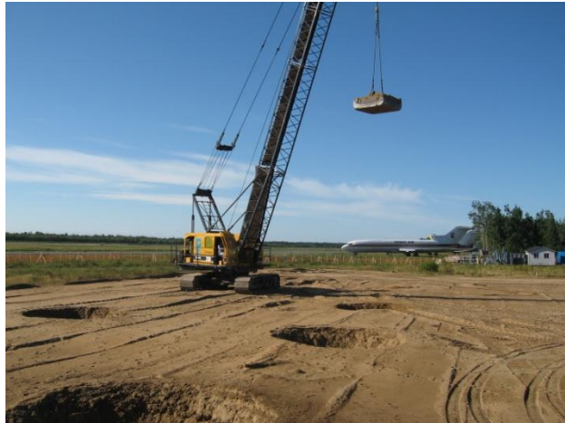
Figure 9. DC crane working away from the building.
