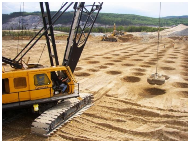
Figure 2. 125 ton capacity crane and 15 tonne tamper used for the Peribonka Dam (Québec) foundation densification.
