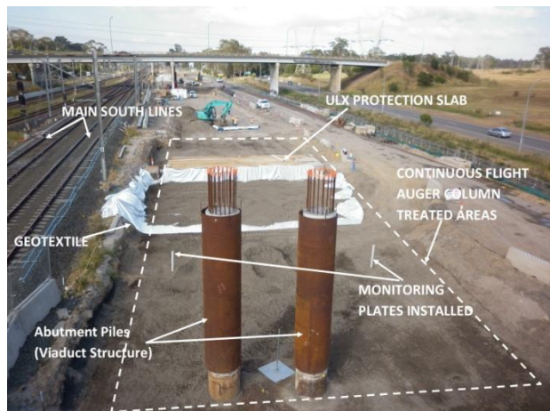
Figure 13. Construction of CFA columns/LTM system under progress
