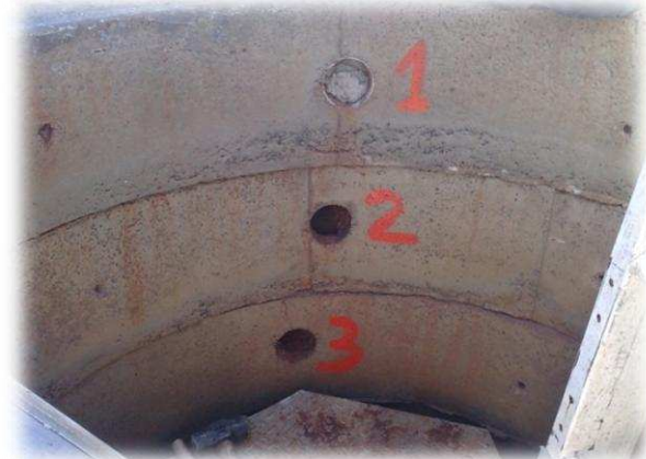
Figure 2. Detail of the holes
