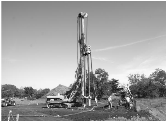
Figure 9 – CMC installation under the MSE Wall
