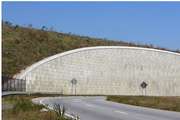
Figure 1 – view of an MSE Wall structure
