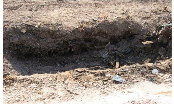
FIGURE 7 Test Pit showing MSW layer
