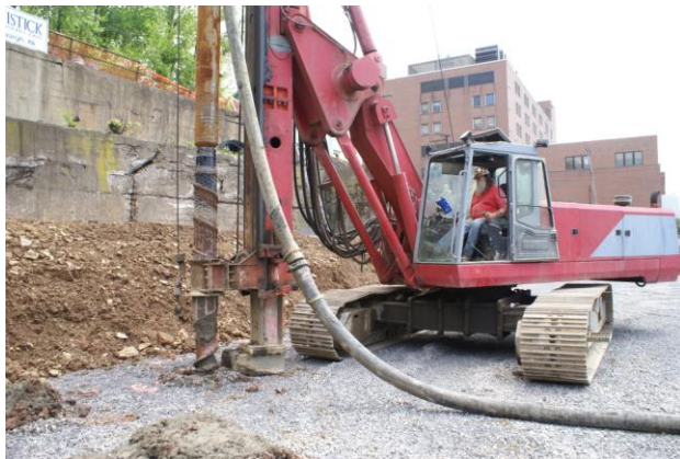
FIGURE 2 Installation of CMCs.
