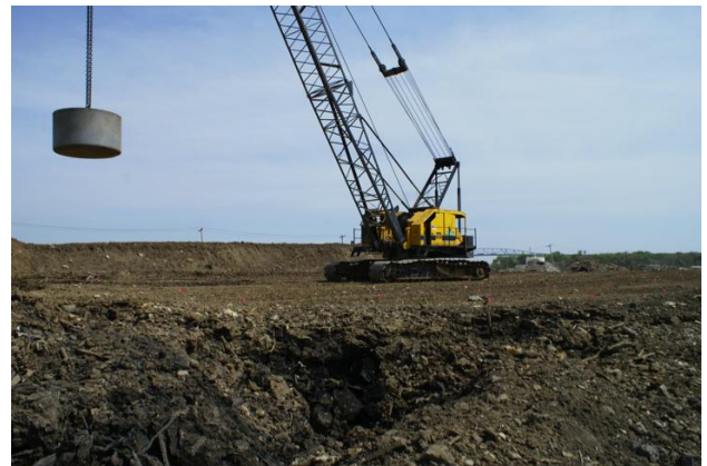
FIGURE 12: Dynamic Compaction Operations
