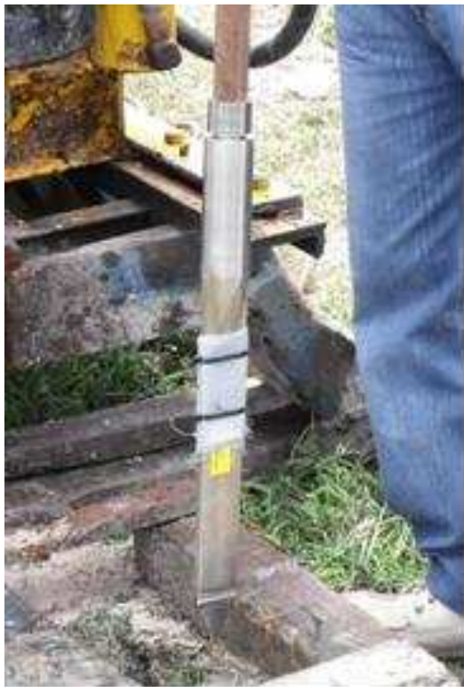
Figure 3. Piezo-cell ready to be driven
