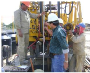
Figure 11. Installation of vibrating wire piezometers
