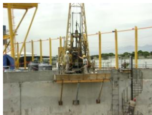
Figure 7. Working platform to install the inclinometers through the diaphragm wall
