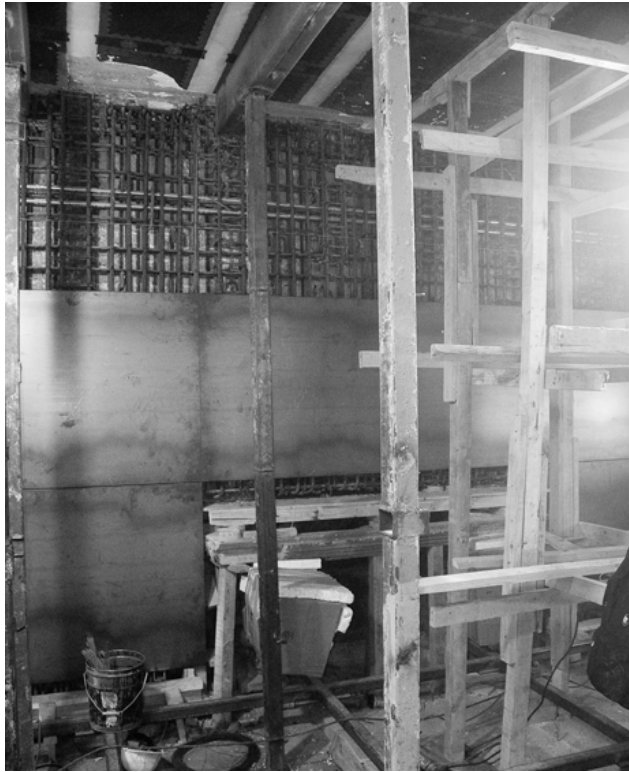
Figure 4. Strengthening of the house with reinforced concrete walls (Courtesy of Fondo Hexa)
