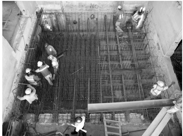
Figure 6. Construction of the ribbed slab for underpinning
