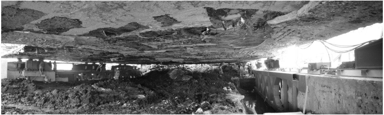
Figure 10. Panoramic view under the house foundation being supported by the hydraulic jacks prior to its moving
